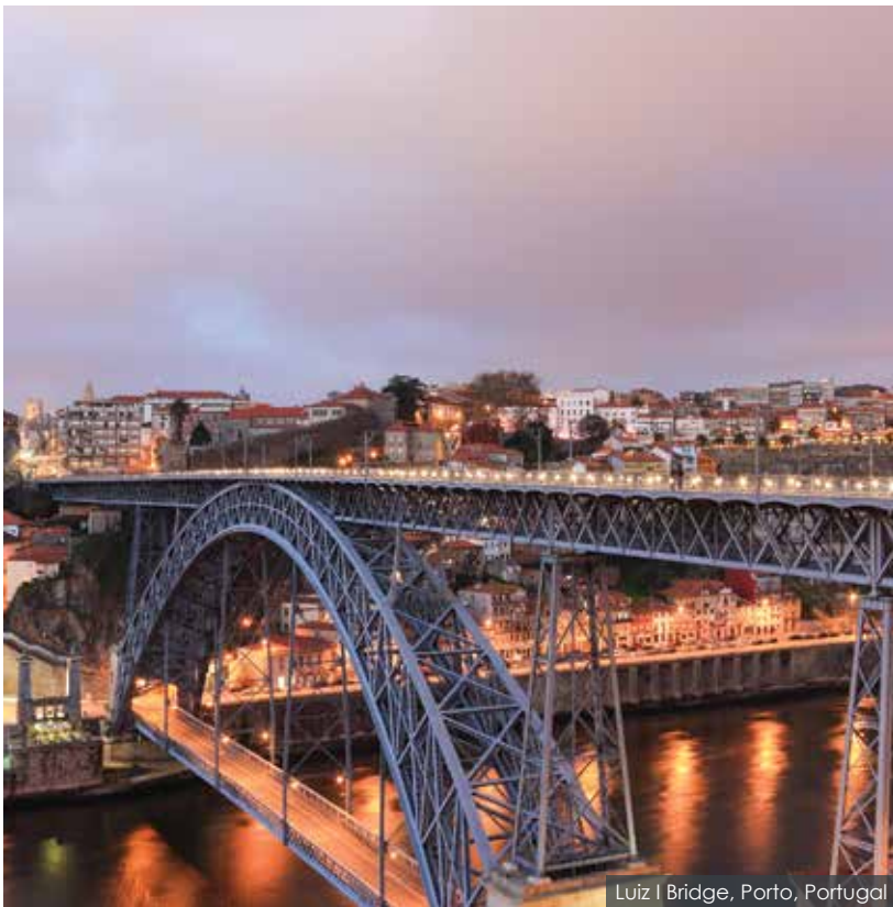
Luiz I Bridge, Porto, Portugal
